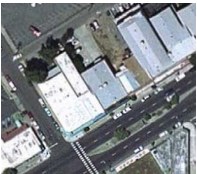
Current North Sacramento-Hagginwood Library Site
